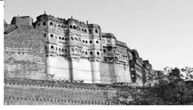
High and strong walls
